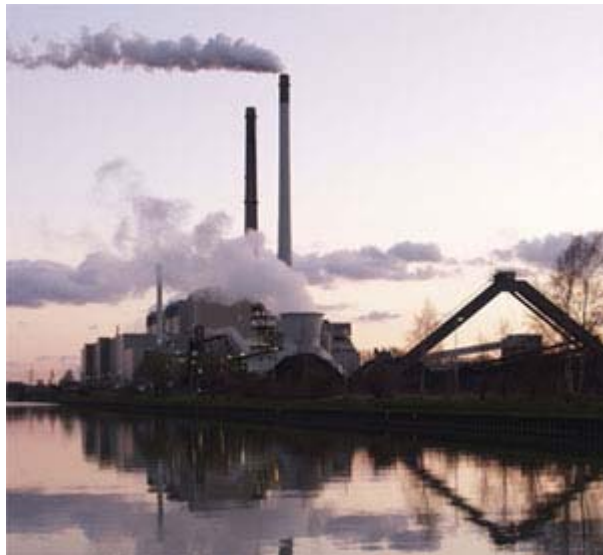
Coal power plant in Datteln, Germany, at the Dortmund-Ems-Kanal. Image by Arnold Paul.
