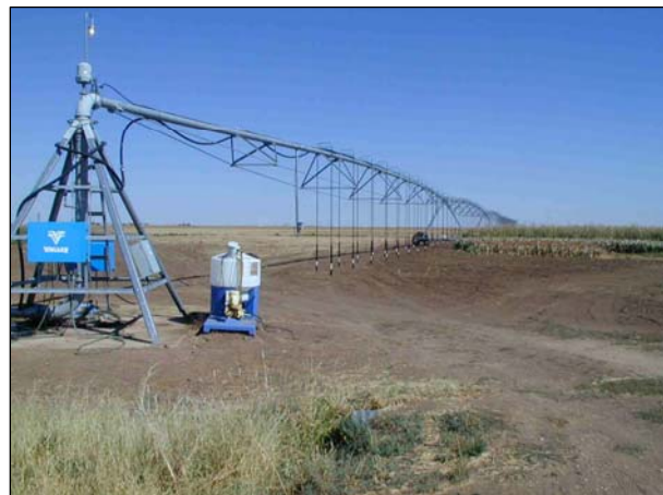
Low Elevation Spray Application (LESA) Center Pivot Irrigation System (Photo: Dr. Clay Robinson)
